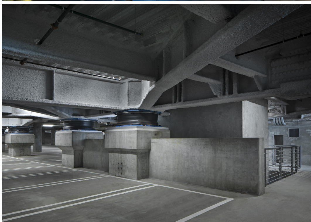
◀ TRIPLE PENDULUM ISOLATOR TESTING, DISPLACEMENT \ ▶ TRANSFER FLOOR FRAMING
