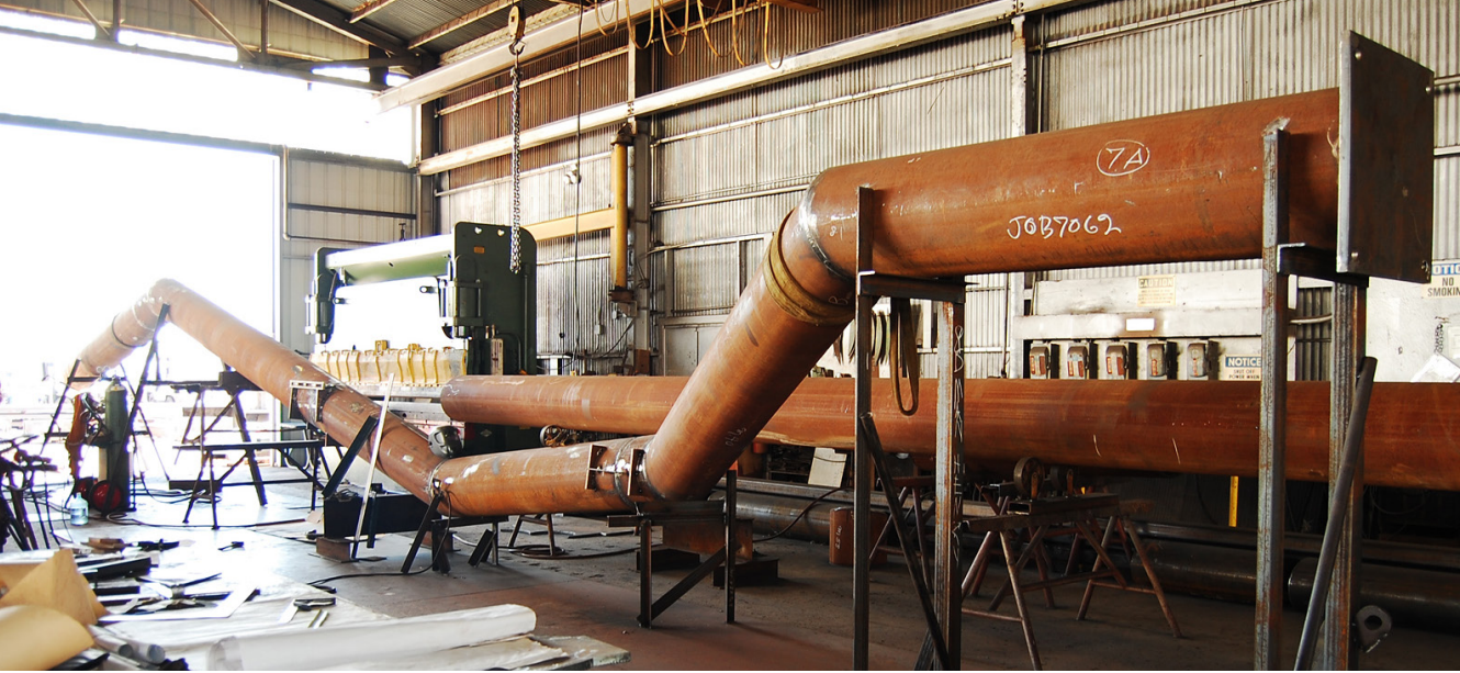
▽ WAFFLE COLUMN STEEL SHOP DRAWING \ ▲ WAFFLE COLUMN FABRICATION
