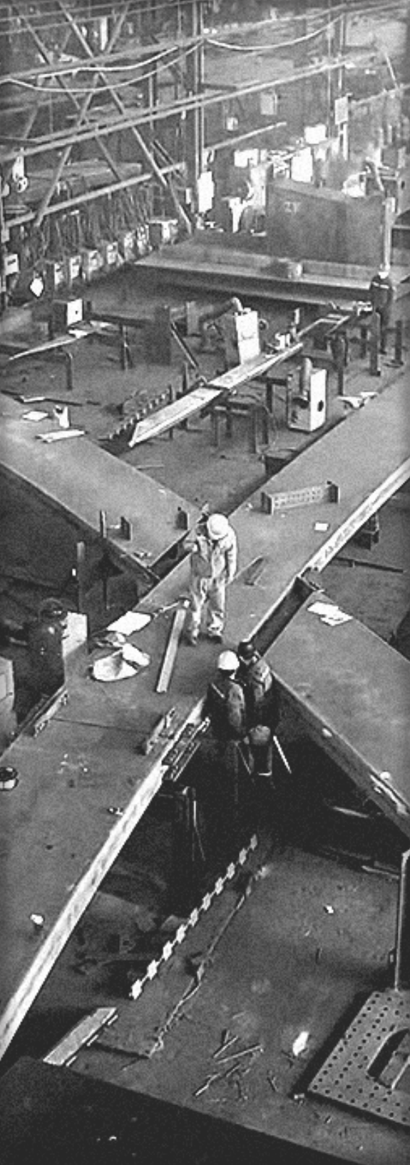
(W)RAPPER BAND FABRICATION, CHINA [COVER: (W)RAPPER STEEL ERECTION]
